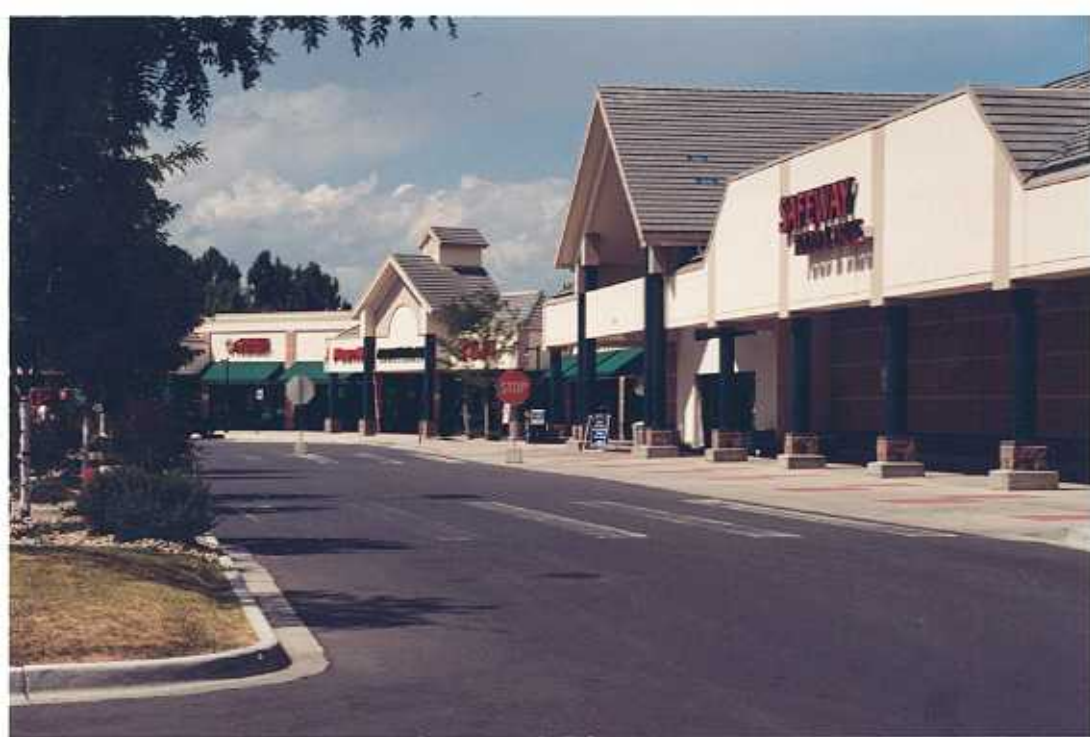
RUBLOFF/SW WILLOW RUN, LLC NEC 128 TH AVENUE AND ZUNI STREET WESTMINSTER, COLORADO
