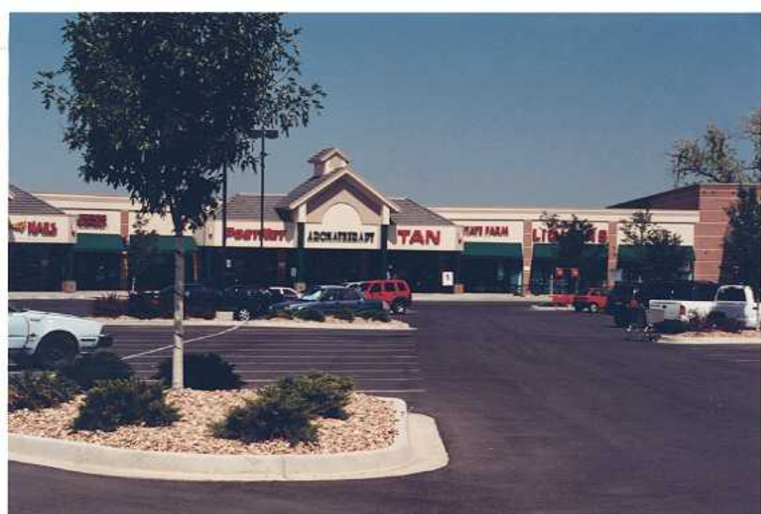
RUBLOFF/SW WILLOW RUN, LLC NEC 128 TH AVENUE AND ZUNI STREET WESTMINSTER, COLORADO
